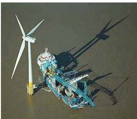
Scroby Sands Wind Farm, Great Yarmouth, Norfolk © English Heritage, NMR ref no NMR 23436/32
